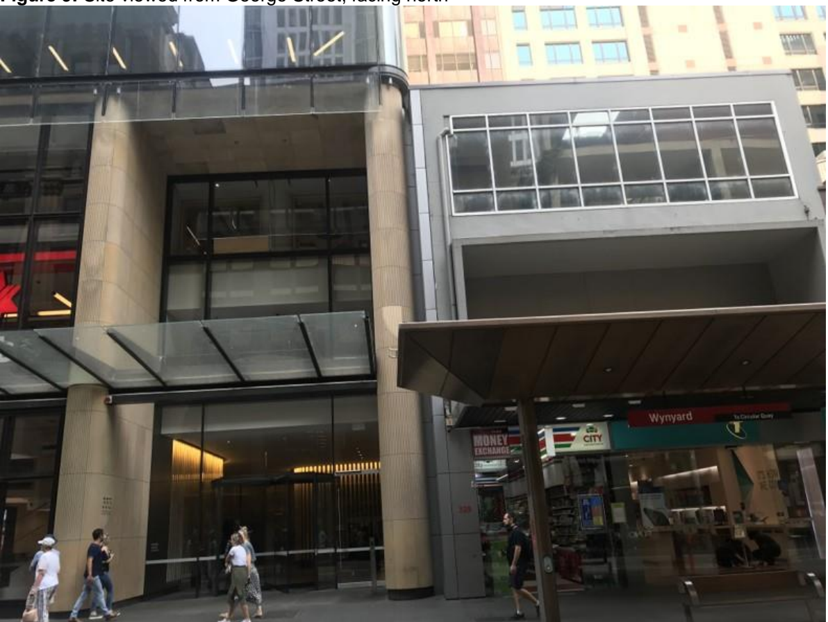
Figure 10: View of 333 George Street and the subject site from George street, facing west
