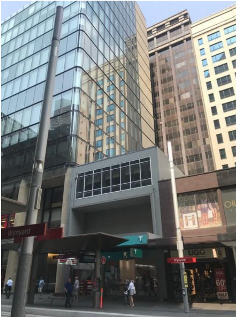
Figure 3: Site viewed from George Street, facing west
